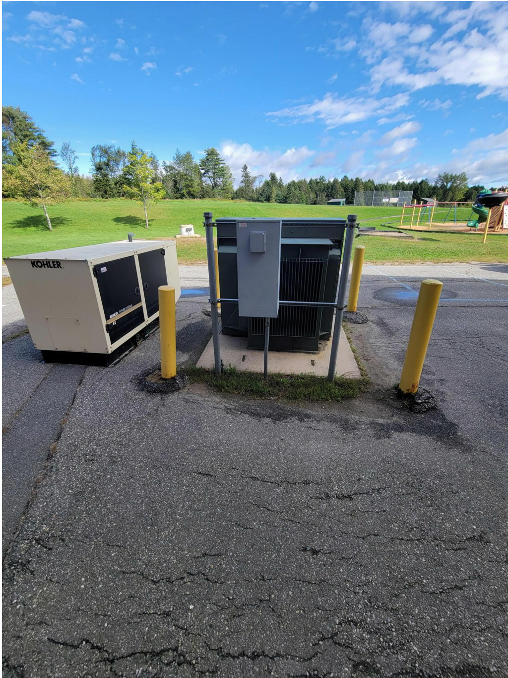
Figure 2 Generator and Transformer Layout
