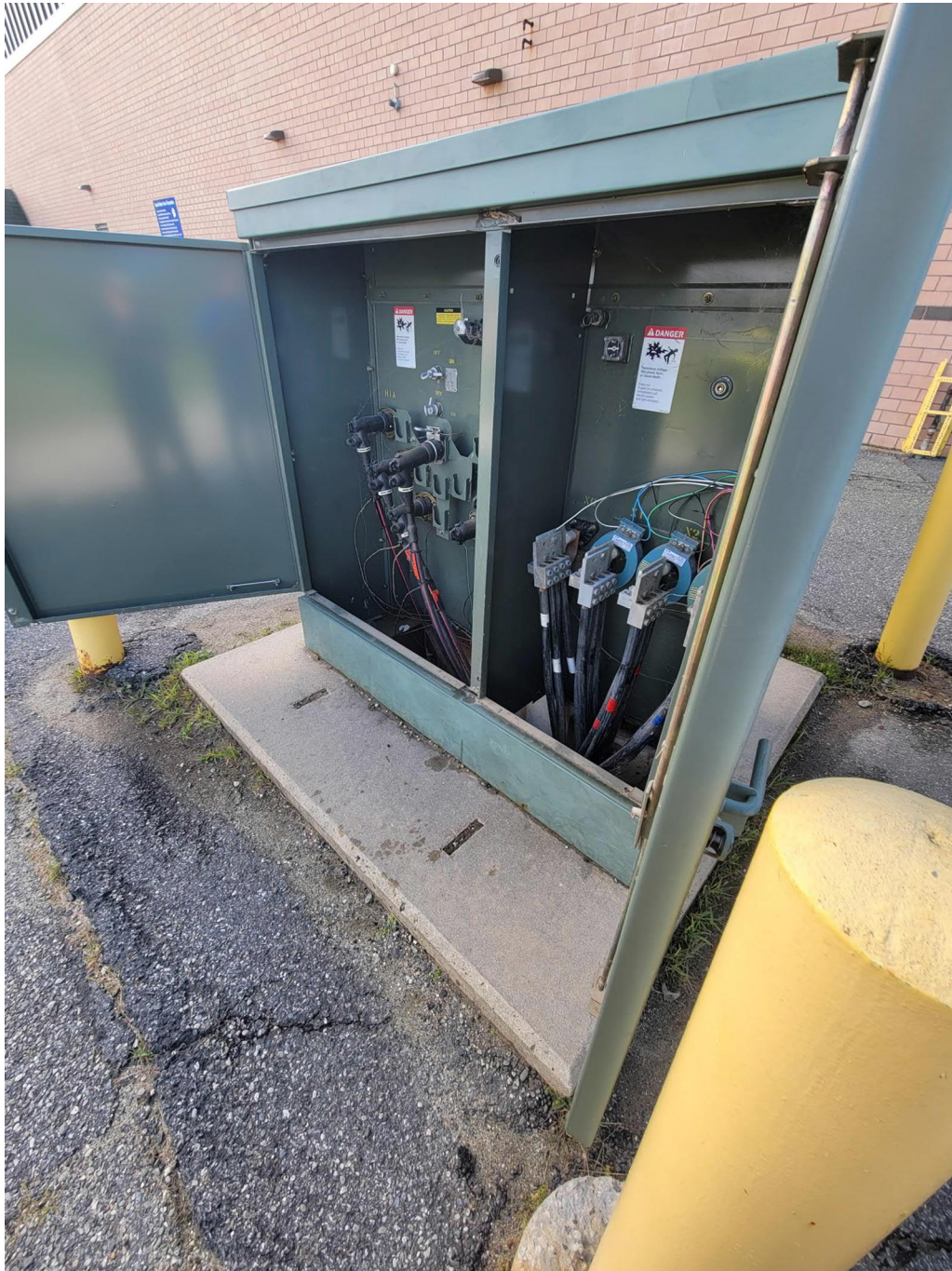
Figure 1 Transformer Interior
